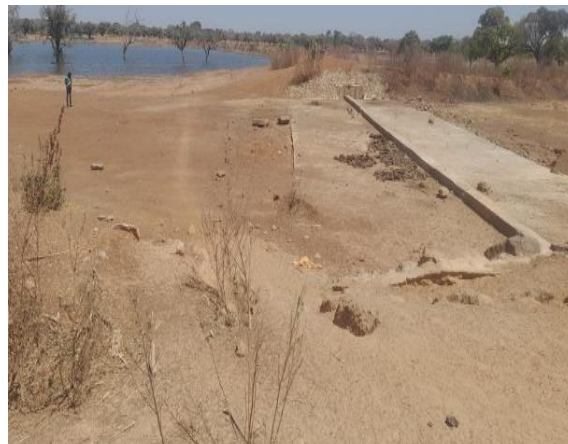
Figure 6: Spillway and High Elevation of the Impounded Area
